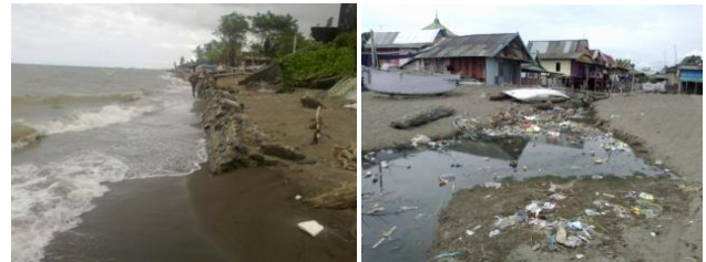
Fig.8. Beaches are experiencing abrasion and environmental conditions of the housing sewer
